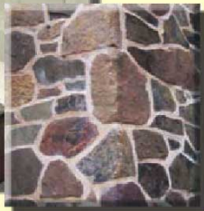
Thin Veneer with L Shaped Corners
